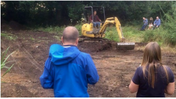
The work progresses - overseen by our friends from Norfolk Rivers Trust
