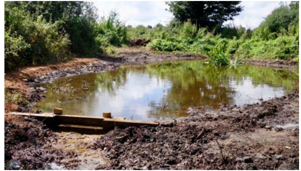
The finished scrape with sluice to slow the flow and encourage biological filtration
