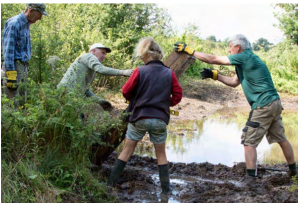
Installing the sluice to help regulate the flow through the system
