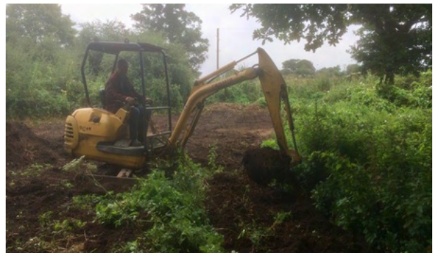
Construction begins by blocking the original channel
